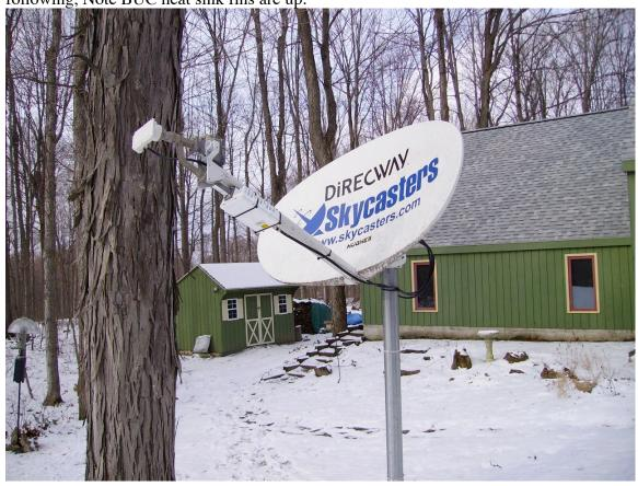
Use tie wraps to secure BUC to feed arm.
