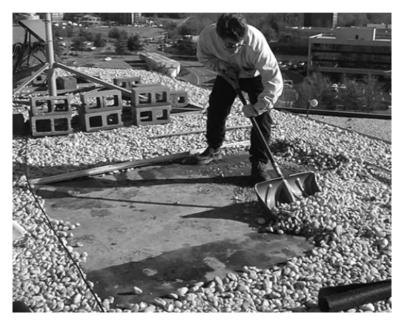
Figure 34: Clearing gravel from the installation location
